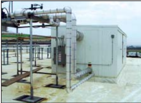
ROOF TOP INSTALLATION
